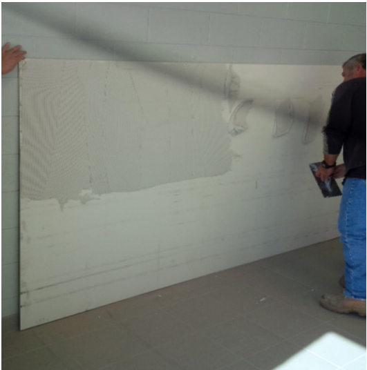
Example of full skim coat being applied
