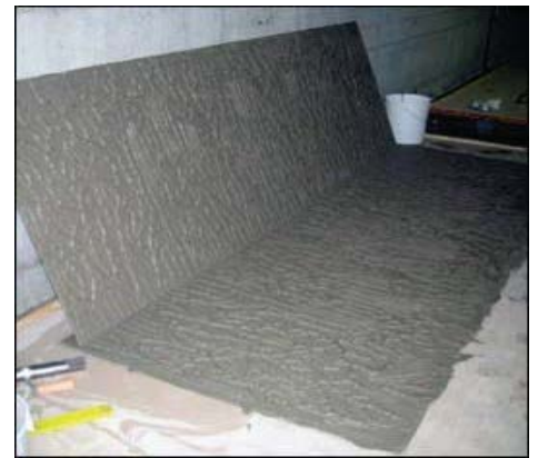
Example of proper full mortar coverage
