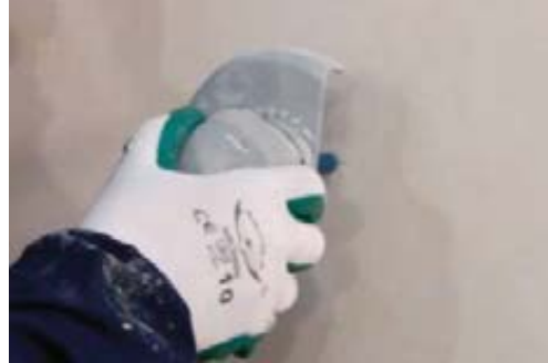
Image shows contact of variable speed grinder with diamond circular bit
