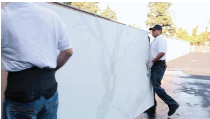
Example of suction cup handle being used. Panel weight is approx. 150 lbs and no more than 2 people are suggested to move
