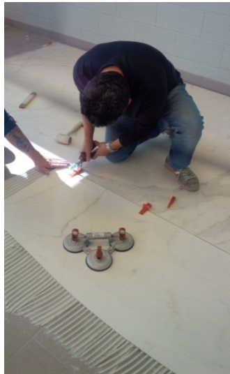
Self-leveling system being used for floor installation
