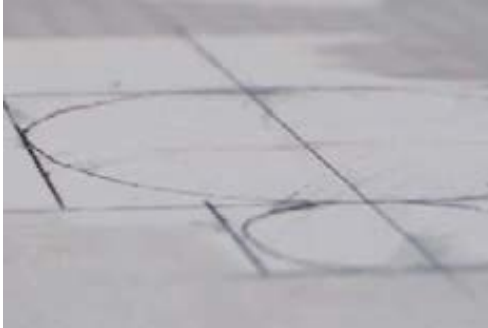
Example of initial drawing for plumbing fixtures cut out
